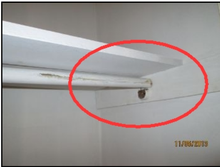
Master Bedroom Closet Clothes Hanging bar improperly installed
