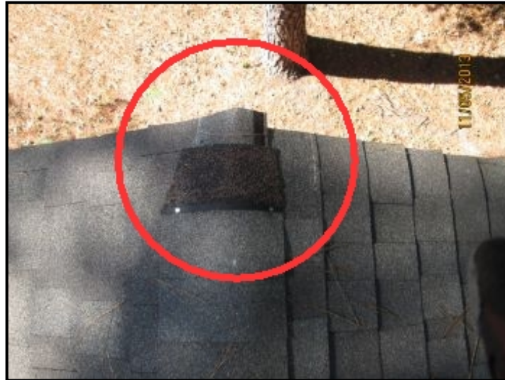
Shingle missing on ridge
