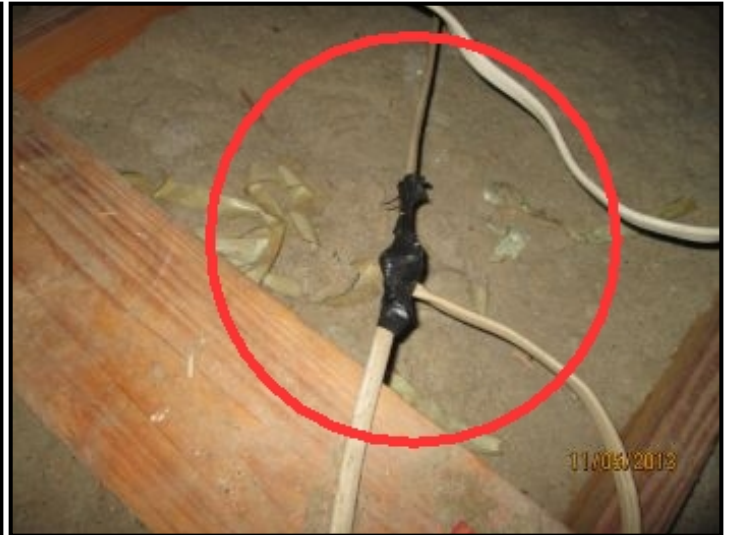
Connections made outside of a Junction Box, which is a potential shock or electrocution hazard.
