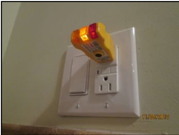
Master Bathroom Upside Down GFCI showing Open Ground (Top)
