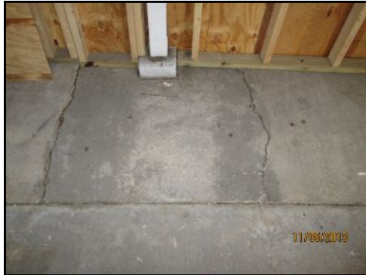
Common cracks noted.
