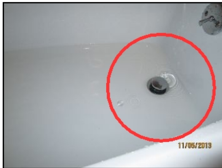
Hall Bath. Drain OPEN but still holding water
