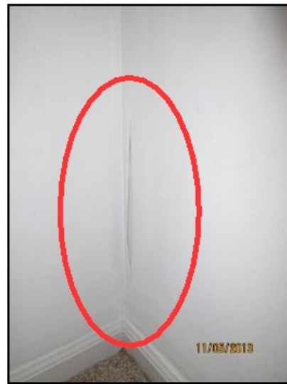
Master Bedroom closet Drywall Tape separation
