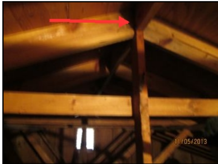
Ridge Beam construction
