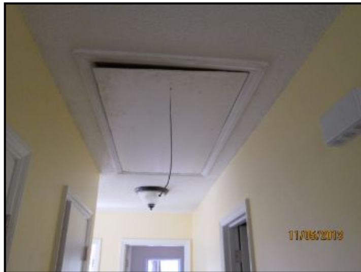
Access Hatch not flush to ceiling
