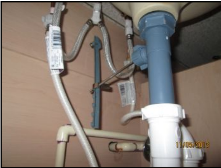
Stopper is missing/inoperable. Both sinks in Master Bedroom. Left sink
