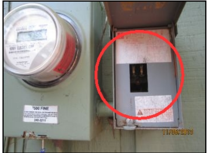
Exterior Breaker box has NO BREAKERS
