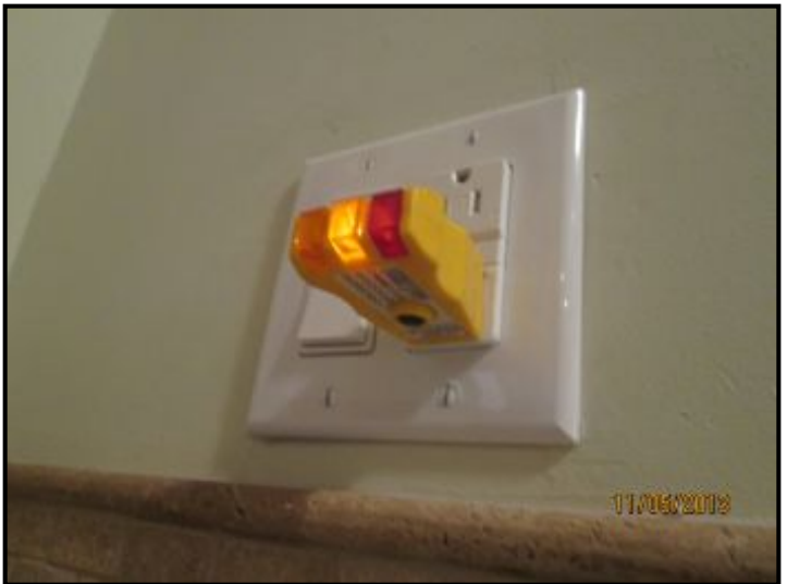
Master Bathroom Upside Down GFCI showing Open Ground (Bottom)
