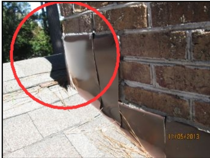
Small portion of the Flashing appears installed improperly; see photo. Recommend repair.
