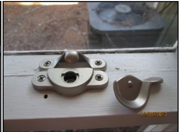
Master Bedroom Window Hardware broken
