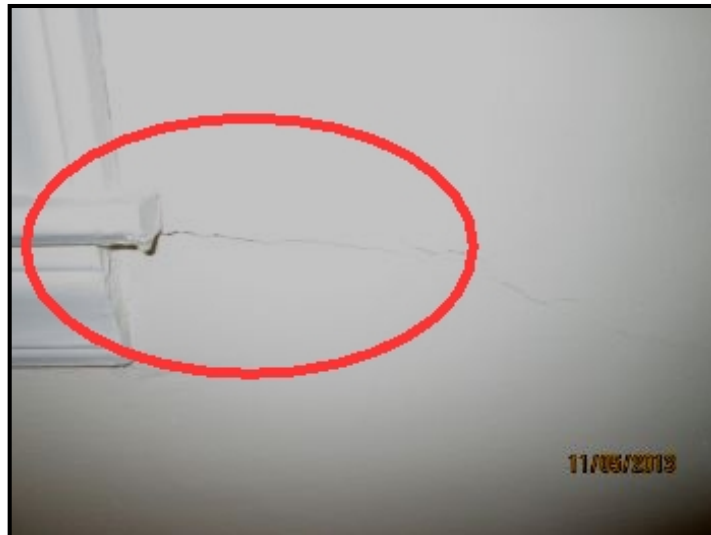
Settlement crack at Master Bedroom window
