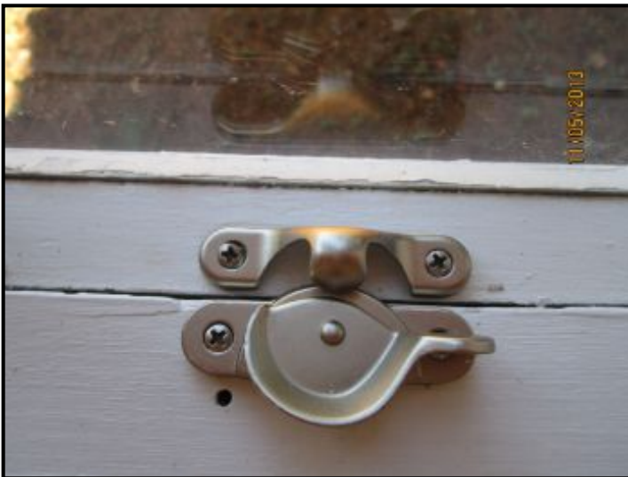
Bedroom #2 Window Hardware needs to be relocated in order for window to be operational
