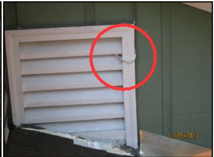
Vent screens noted as functional. Although Coaxial cable noted to be pushed through South side vent.
