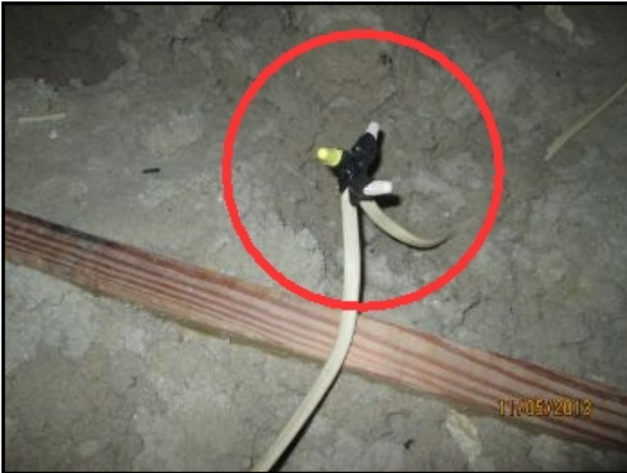
Wire ends are outside of a Junction Box, which is a potential shock or electrocution hazard.
