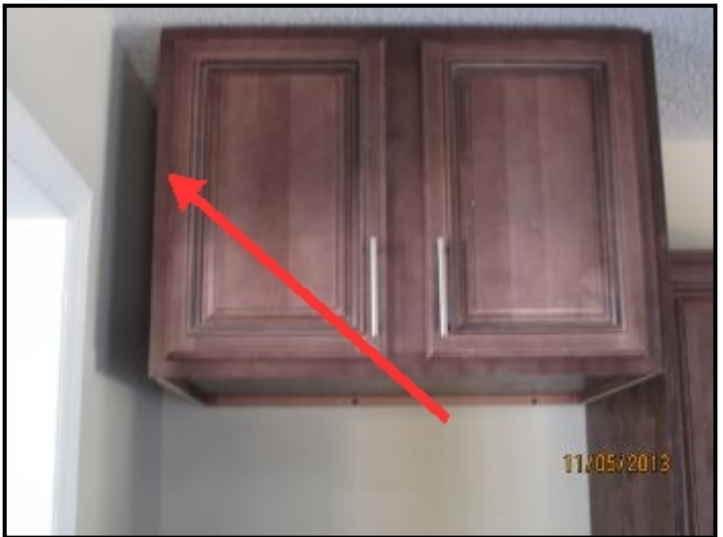
Filler/Spacer missing
