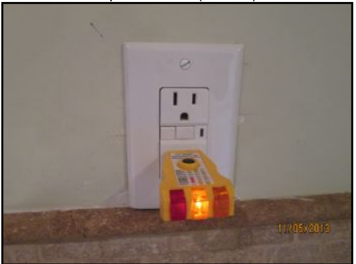
Master Bedroom Opposite GFCI also showing Open Ground
